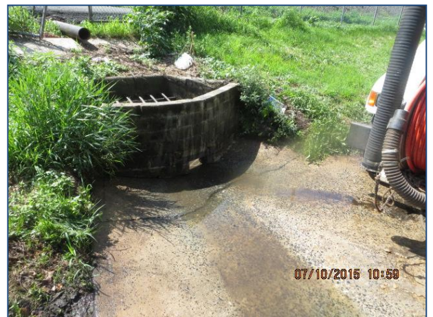
Cleaning the Walnut Street Basin. The jet-vac truck vacuumed out the leaves and debris, which would have restricted flow of stormwater. When Roselle Park puts the camera truck into service, it will be able to view the lines to see if there are any obstructions, and clear them to alleviate future flooding.
