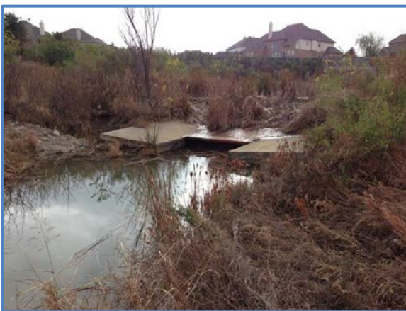
Care and maintenance of retention areas within Grand Prairie, Texas, allow stormwater and flood waters to be stored and released more slowly into the drainage system. At left: an overgrown and clogged channel. At right: the same area after proper maintenance.
