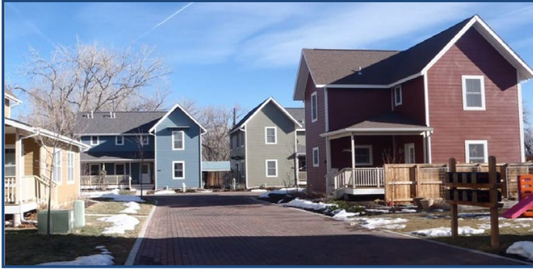
Photo 1. The Toby Lane Development in Boulder was protected from flood damage in September 2013 because the homes were elevated two feet above the 100-year flood elevation.
