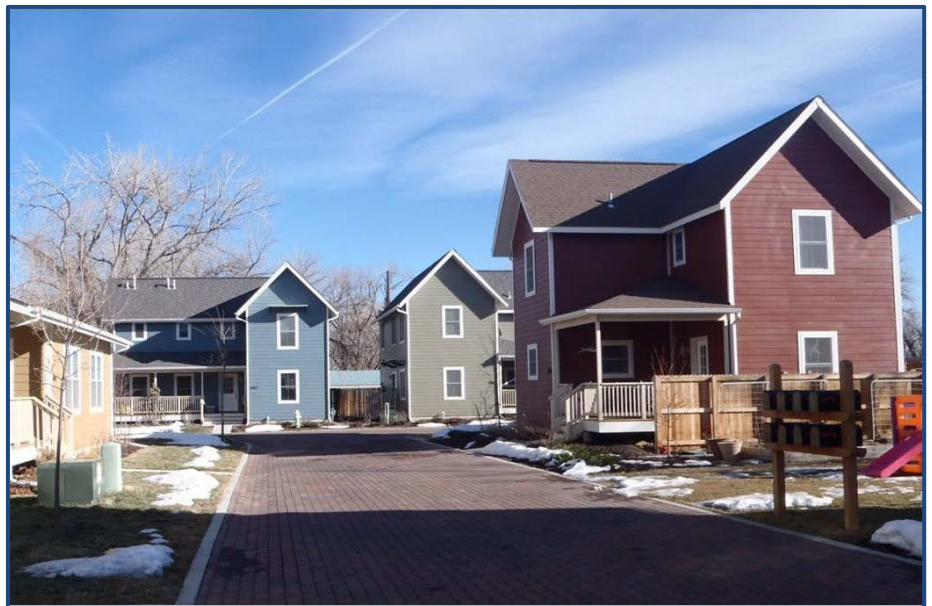
The Toby Lane Development in Boulder, Colorado, remained undamaged in the 2013 flood because the homes were elevated 2 feet above the base flood elevation.
