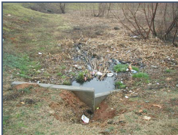
Growth and headwall erosion show a lack of maintenance in this private retention basin.
