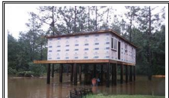
Construction on elevated flow-through foundations is much less disruptive than filling a building site, as shown by this structure in Baldwin County, Alabama.
